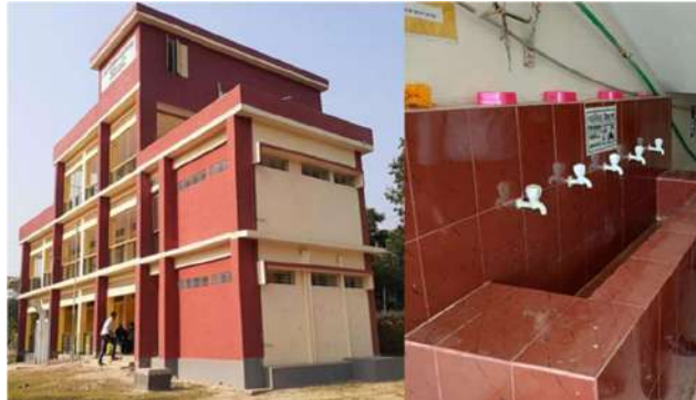
Fig. 10 (L): Constructed Wash Block (R): 5 outlet water collection basin
